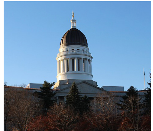
Maine State House in Augusta
